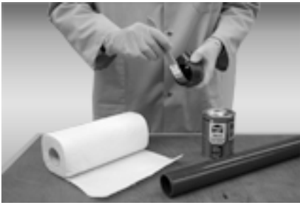
Applying the cement
