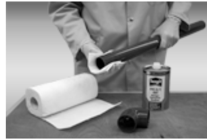
Cleaning the pipe and socket
