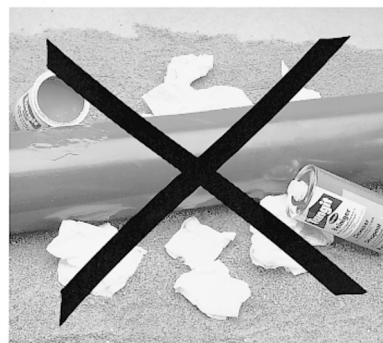
The pipe trench is not a rubbish tip
